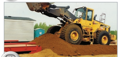
3 Backfill to bulkheads and finish ramps.
